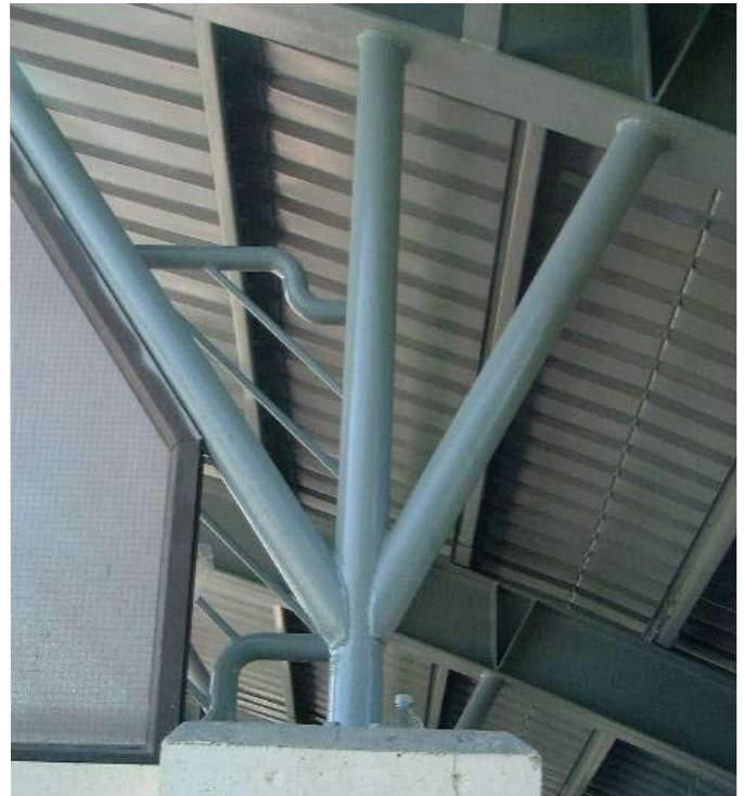
STANCHION AFTER RECEIVING THE BELZONA TREATMENT
